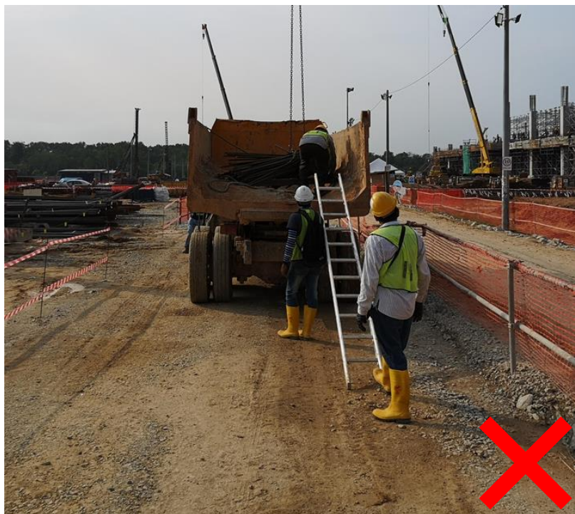
Unsafe: Vertical ladder used in inclined position for access to vehicle
