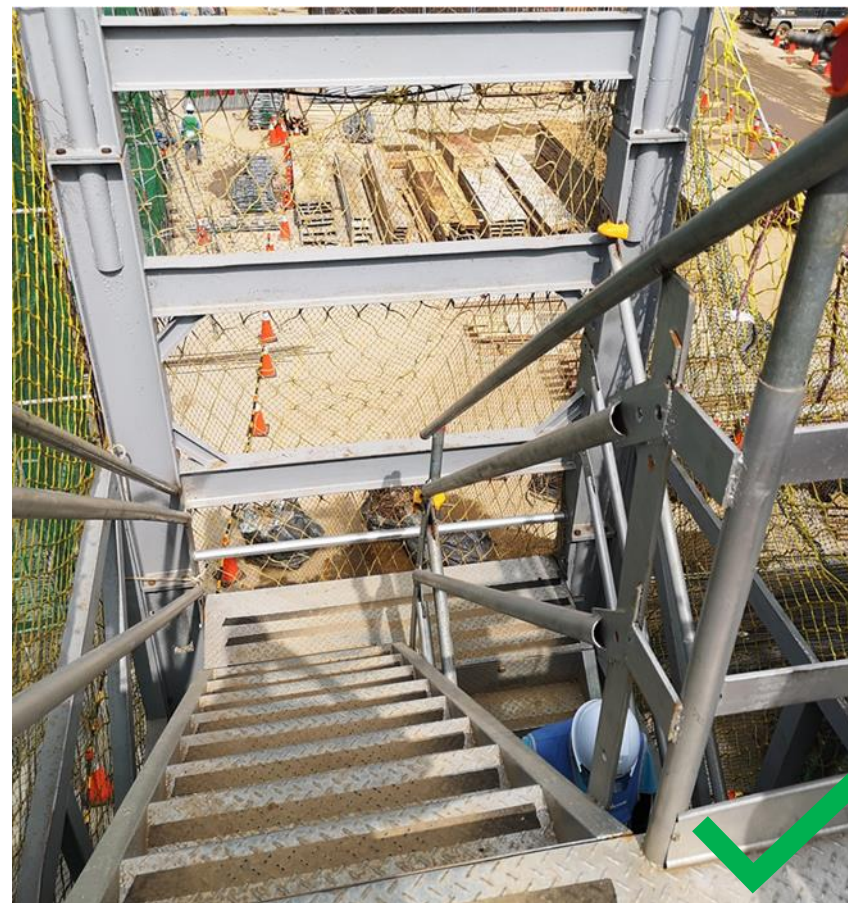
Best Practice: Provide proper temporary stairway access to work areas
