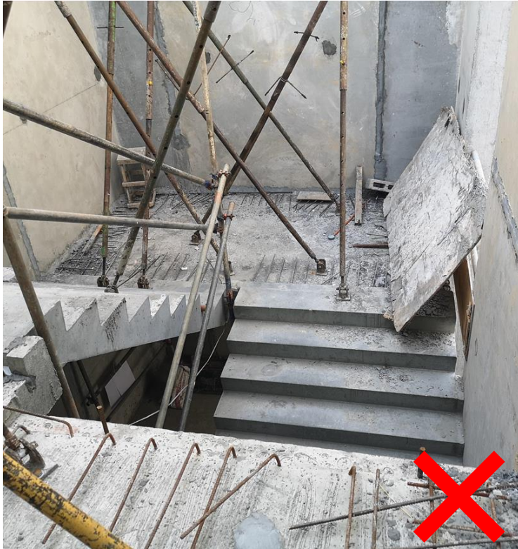
Unsafe: Stairway open for use without guardrails and tripping hazards
