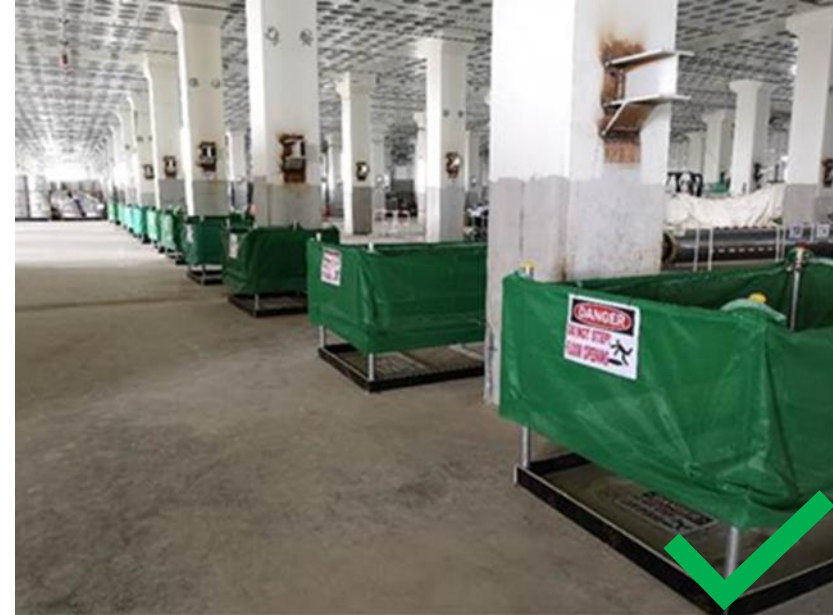
Best Practice: Hole opening with guardrails, cover, toe-board and danger notice
