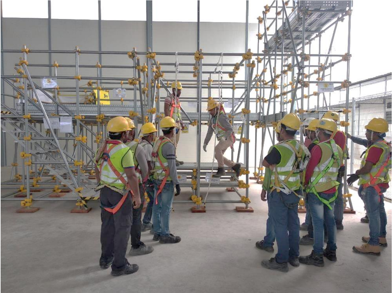
Training scaffolding module with access and working platform for Working at Height and Rescue training and exercise
