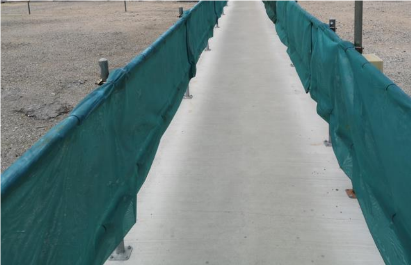
Drainage system mockup to prevent environmental pollution into public drainage system and designated safe walkway
