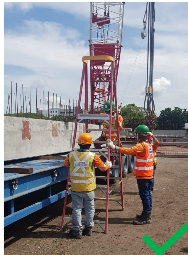
Best Practice: Use proper platform ladder or similar for access to vehicle
