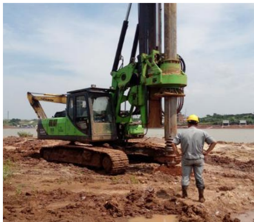
Hydraulic Rotary Piling
